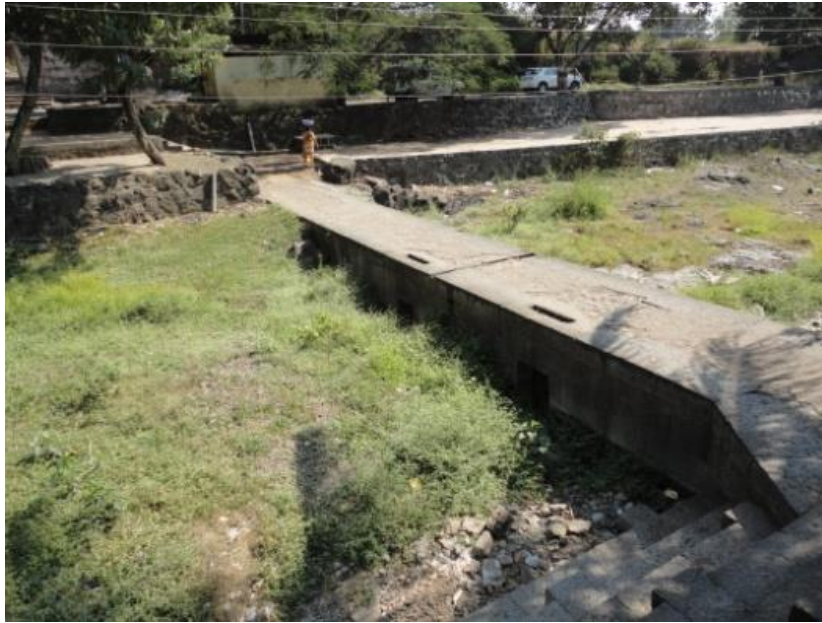
Figure 5: Embankment at Hiware
